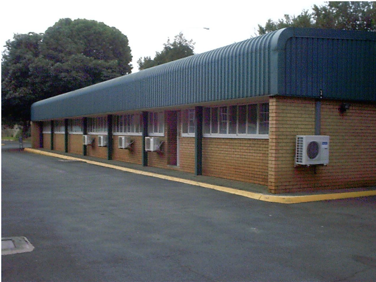
Self-Contained Self-Rescuer Testing Facility, Johannesburg, South Africa
